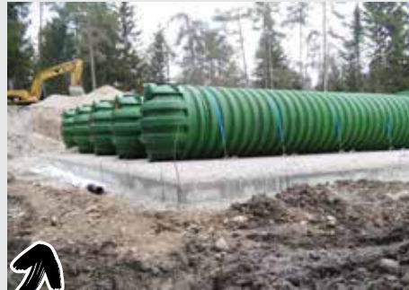
Installation of products and hand over the required technical documentation
