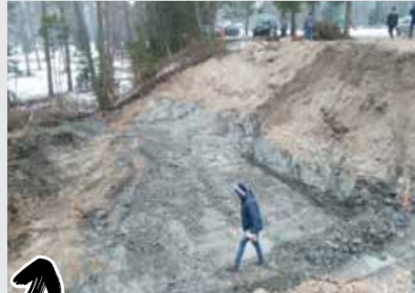
Visit the construction site
