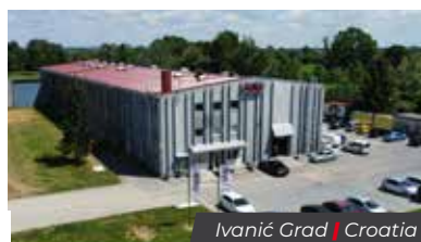
Roto Group Headquarters
